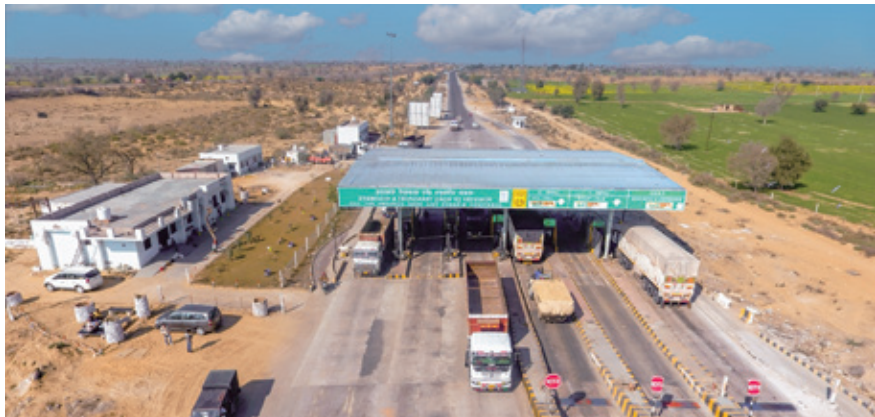
Roads and highways infrastructure - Construction projects
