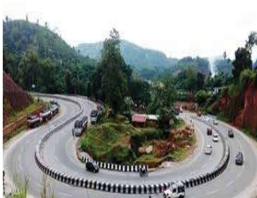
ROADS & HIGHWAYS – CONSTRUCTION/EPC
