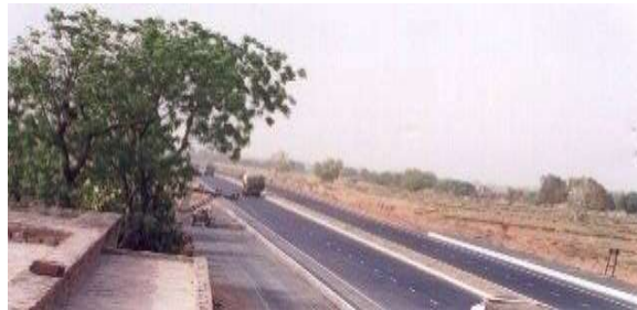
4 lane of km 41-51 of Agra Dholpur of NH-46 (earlier NH 3), in the state of Rajasthan
