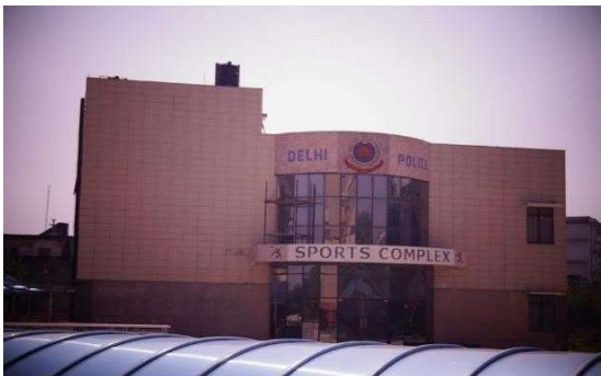
Police Station & Residential Quarters at Kondli, New Delhi for MHA, Delhi Police through RITES Ltd.
