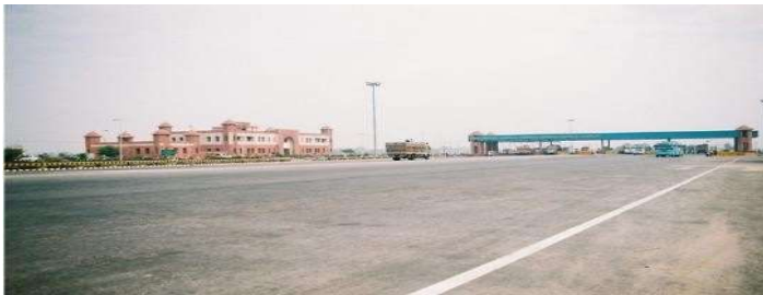
Toll Plaza construction at Delhi –Agra, NH-44 (earlier NH-2)
