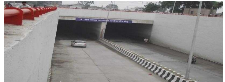
Construction of RUB at Badli, New Delhi
