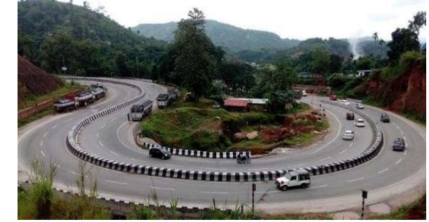
Widening & Strengthening of existing National Highway from 2 lane to 4 lane of Sonapur to Guwahati section of NH-115 (earlier NH 37)
