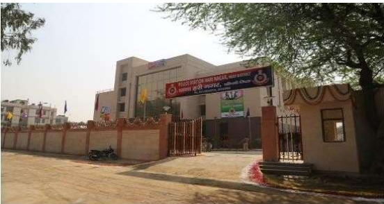
Construction of Police station & Residential Quarters, Hari Nagar, Delhi for MHA, Delhi Police through RITES Ltd.
