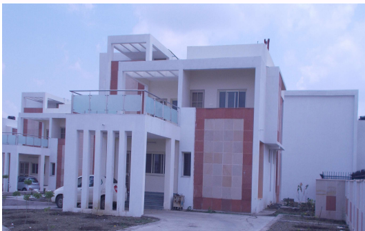
Construction of Director, Dean Bungalow, QIP Centre & Accommodation for School of Planning & Architecture at Bhopal
