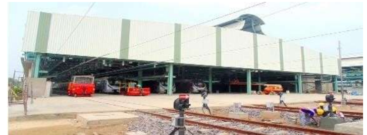
Construction of Metro rail depot, Kalindi Kunj, New Delhi
