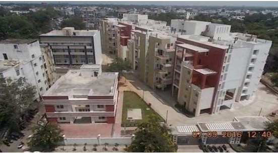
Construction of 92 flats at Mahadev Towers, Bhopal for MP Housing & Infrastructure Development Board
