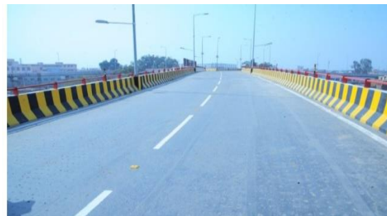
Construction of 2 lanes at Sonapat
