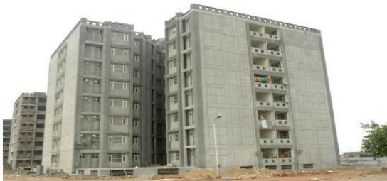
Construction of Police station & staff flats, New Delhi
